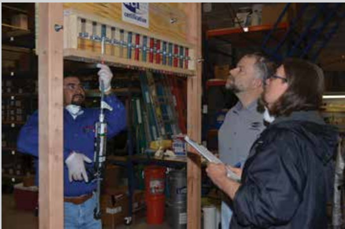
ACI's Adhesive Anchor Installation Inspector certification provides an understanding of what an adhesive anchor installer should—and should not—be doing, such as this example of a poorly installed anchor (right)
