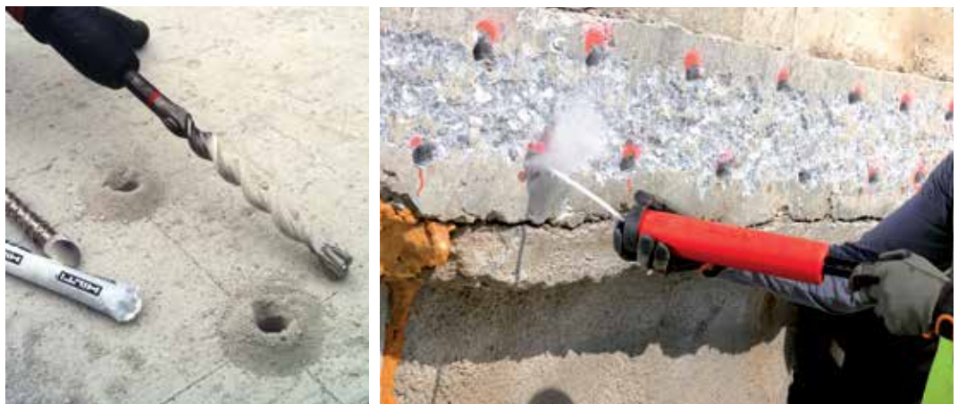
Fig. 1: Adhesive anchors are installed in holes drilled in hardened concrete. Critical installation steps include cleaning the hole in accordance with the manufacturer's installation instructions (MPII) and, for injection systems, injecting the adhesive. OSHA requirements for controlling exposure to silica dust must be observed
