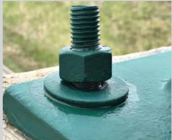
ACI's Adhesive Anchor Installation Inspector certification provides an understanding of what an adhesive anchor installer should—and should not—be doing, such as this example of a poorly installed anchor (right)
