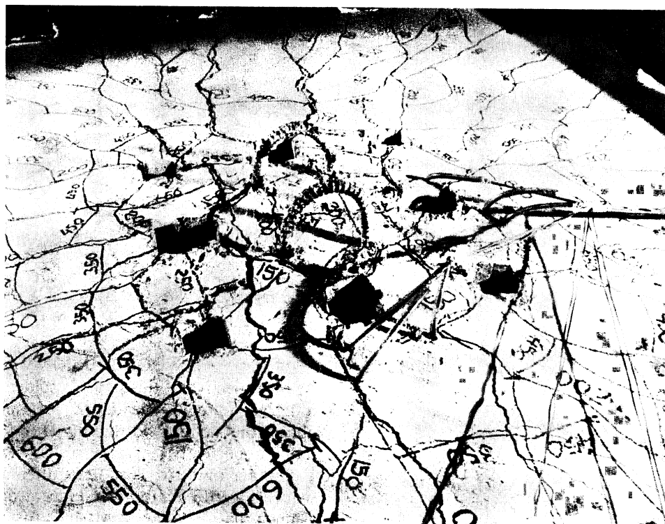
Fig. 13—Specimen 8. Close-up of cracks in the column region
