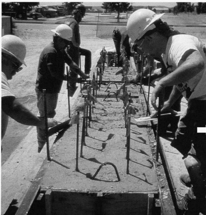
Fig. 6. Completion of casting and finishing pull-out test blocks (May 17, 1996).
