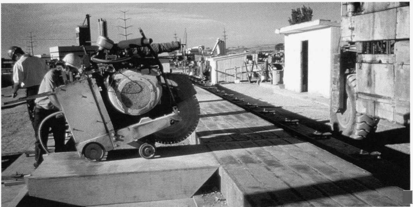
Fig. 14. Release of prestress force by saw-cutting at ends of each 18 ft (5.49 m) beam length (May 18, 1996).
