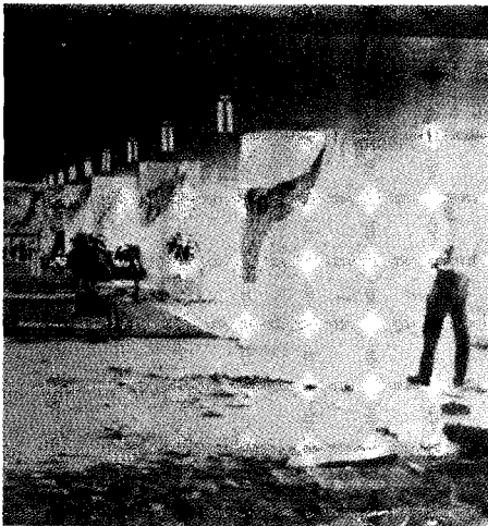
(b) View of failed columns at mezzanine level
