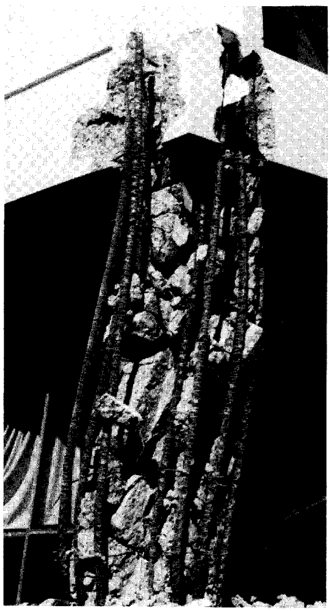
(b) Shattered column with inadequate tie reinforcement
