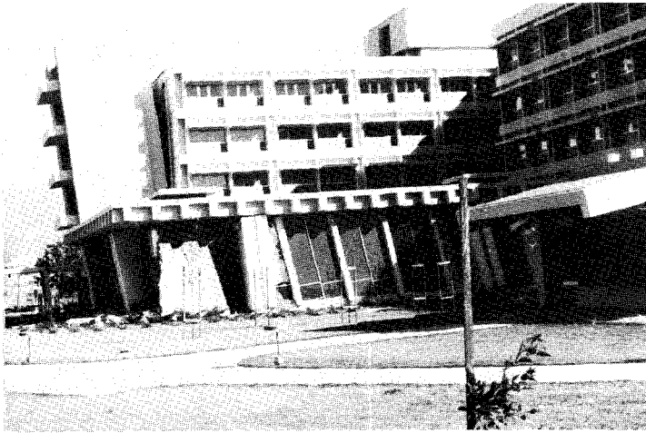
Figure 3 - Olive View Hospital following the 1971 San Fernando Earthquake
