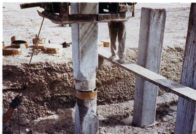
Fig. 2.13. Connector ring pile splice.
