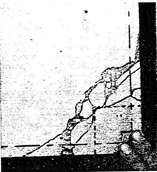
(b) Close up of punching failure at Column 16. Note the exposed reinforcing bars.
