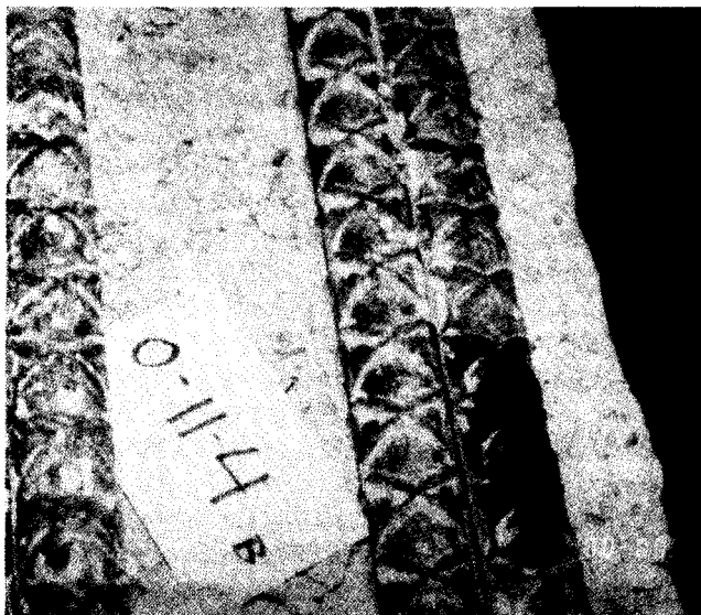
Fig. 5—Appearance of concrete cover and uncoated bars after test
