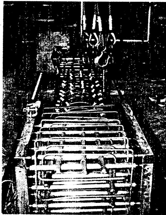
Fig. 2.11: Reinforcing cage placed in the prefabricated steel form.
