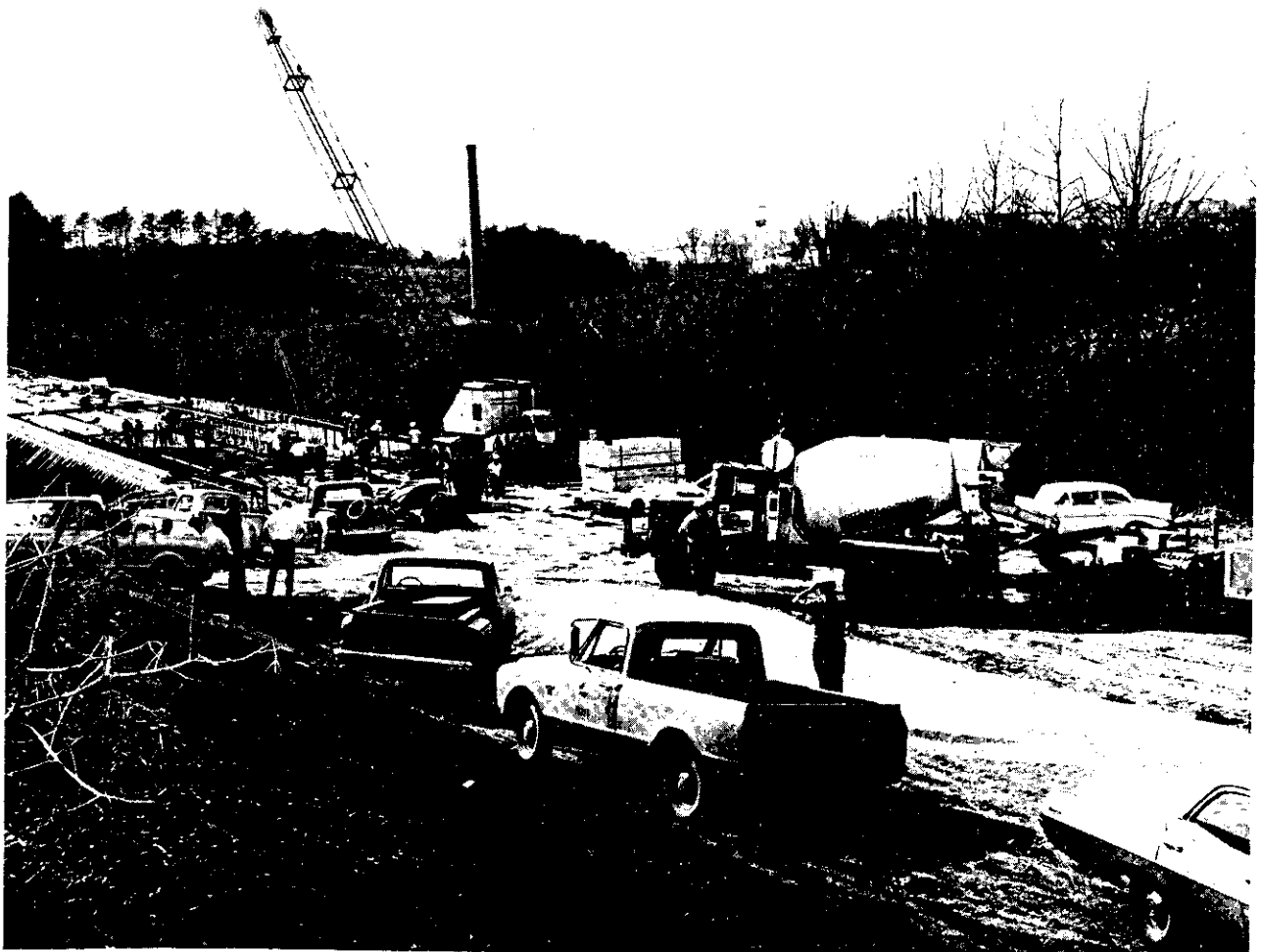
Figure 1. General view of construction area and quipment.
