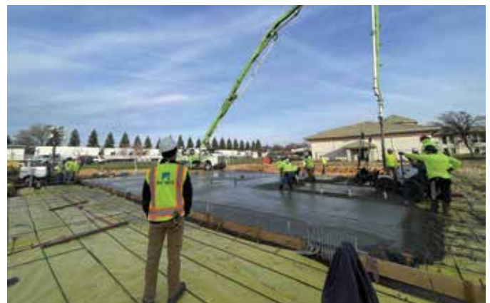
Phase 2 of the Simpson University Business, Technology, and Engineering Building project
