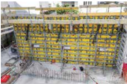
Doka promotes sustainable construction practices, such as heated formwork that facilitates the use of carbon dioxide (CO 2 )-reduced concrete (photo courtesy of Doka)
