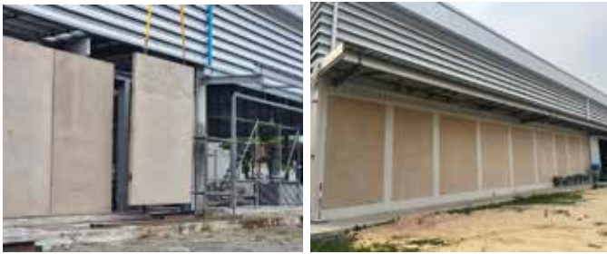
Fig. 8: Installation of a decorative façade made of LC3 concrete
