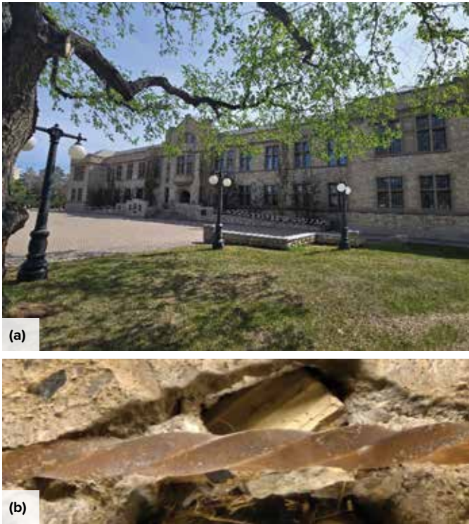
Fig. 3: Peter McKinnon Building on the University of Saskatchewan campus: (a) overview; and (b) inspection port showing twisted square bar reinforcing the main floor slab (photos courtesy of L.R. Feldman)
