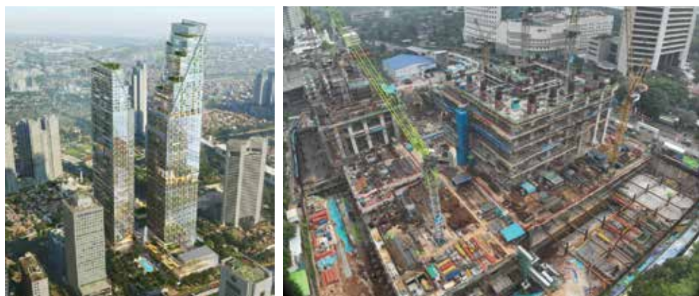
Fig. 7: Concept sketch of The Two Sudirman complex (left), showing the planned 331 m (1086 ft) mixed-use tower and 276 m (906 ft) residential tower, alongside construction 8% progress as of September 2025 (right) (image and photo courtesy of the Mitsubishi Estate Indonesia)
