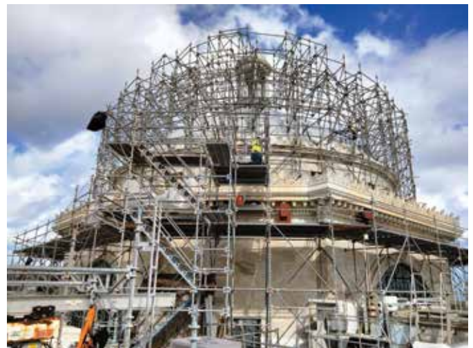
Capitol of Puerto Rico Dome during restoration
