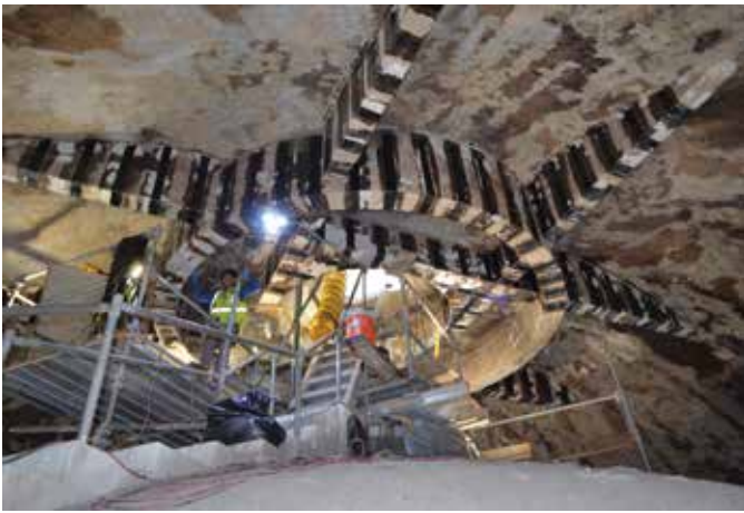
Strengthening with carbon-fiber laminates
