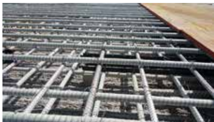
Tied reinforcing bar grid (photo courtesy of Mateenbar Composite Reinforcements)
