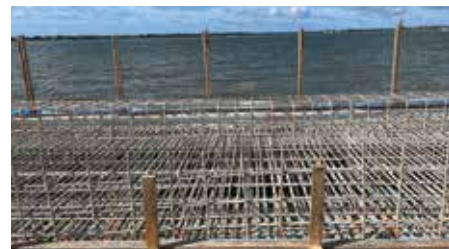
Low Battery Seawall Project in Charleston, SC, USA (photo courtesy of Mateenbar Composite Reinforcements)
