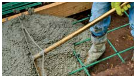
Placing concrete with GFRP reinforcing bars (photo courtesy of Mateenbar Composite Reinforcements)
