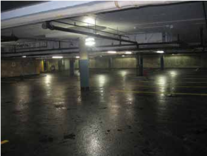
Fig. 4: An underground parking structure with waterproofing
