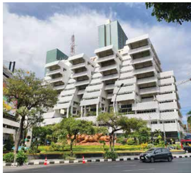
Fig. 5: Wisma Dharmala (Intiland Tower), Surabaya —Completed in 1997, this 12-story office tower by Benjamin Gideon & Associates, with architect Paul Rudolph, was designed under SK SNI T-15-1991-03 11 combining ACI concrete testing and New Zealand seismic detailing. Though it used 90-degree hooks and wider stirrup spacing, the structure followed capacity design principles within a reinforced concrete frame adapted to Surabaya's tropical climate, featuring natural ventilation and sun-shading. Paul Rudolph also designed Wisma Dharmala (Intiland Tower), Jakarta, in the mid-1980s with PT Wiratman & Associates, a tropical modernist landmark known for its stepped terraces, shaded atriums, and bold geometric form that redefined the high-rise design in the capital ( photo courtesy of Josia Irwan Rastandi )
