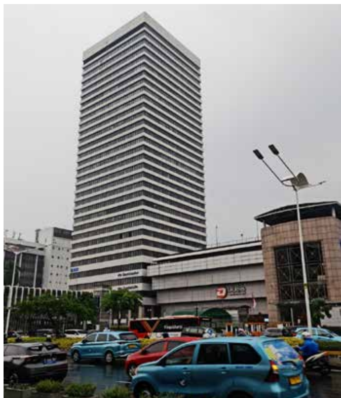
Fig. 4: Ratu Plaza, Jakarta —One of the earliest high-rise applications of PBI 1971, 2 designed by PT Wiratman & Associates. The project integrated ACI and VB standards and employed a tube-in-tube system (perimeter columns resisting lateral loads, a central core carrying vertical loads, and a prestressed flat slab linking them), enabling column-free interiors and improving earthquake vibration dissipation ( photo courtesy of Josia Irwan Rastandi )
