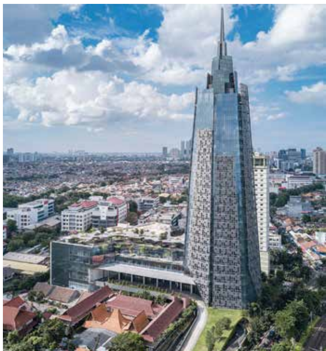
Fig. 6: Kompas Multimedia Towers, Jakarta—Structural design by PT Davy Sukamta & Partners under SNI 03-2847-2013 16 (ACI 318M-11 17 ). This 25-story building with a three-level basement has a gross building area of approximately 57,000 m 2 (68,000 yd 2 ), completed in 2017. This modern development deploys a reinforced concrete core wall and open-frame structural system on bored pile foundations, optimizing resistance to both seismic and wind forces (photo courtesy of PT Davy Sukamta & Partners)
