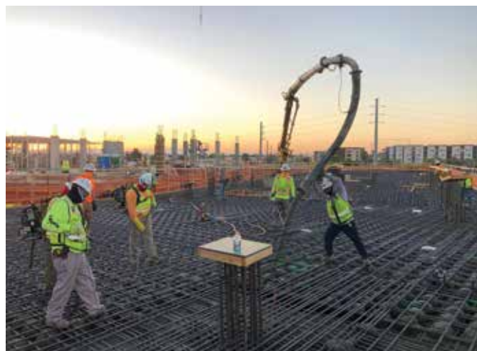
Fig. 3: The voided form installation and concrete placement for the elevated deck (courtesy of McCarthy Building Companies)
