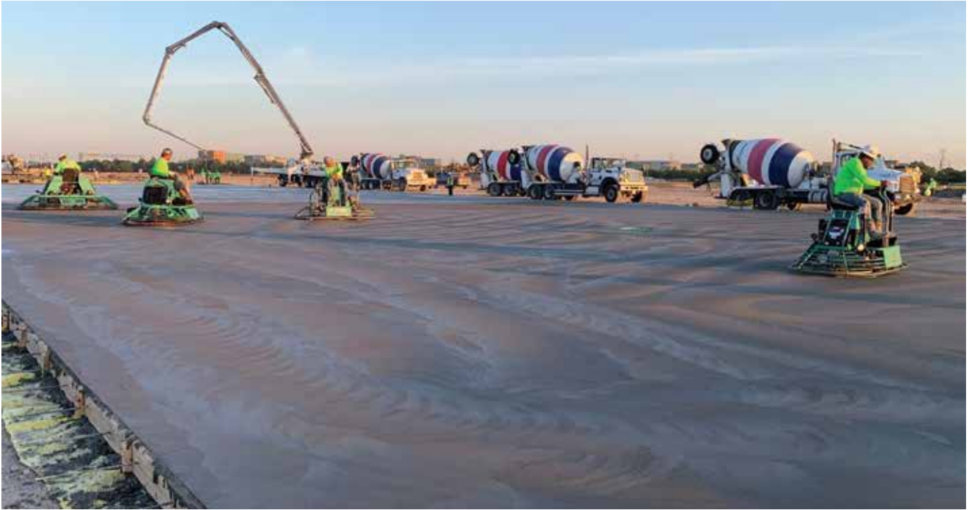
Placement and finishing of a PLC (Type IL cement) concrete slab
