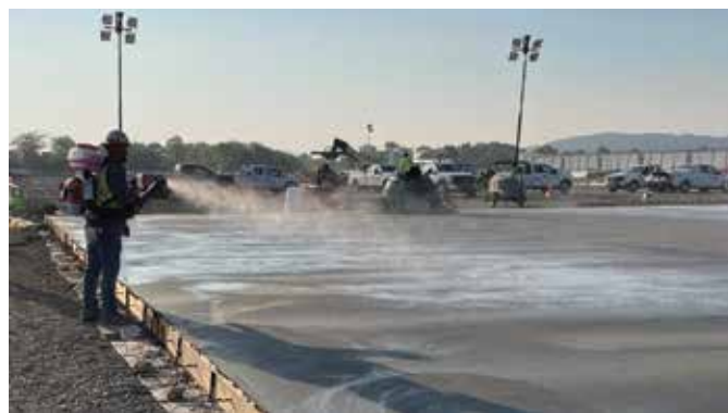
Application of an evaporation retardant on a PLC (Type IL cement) concrete slab
