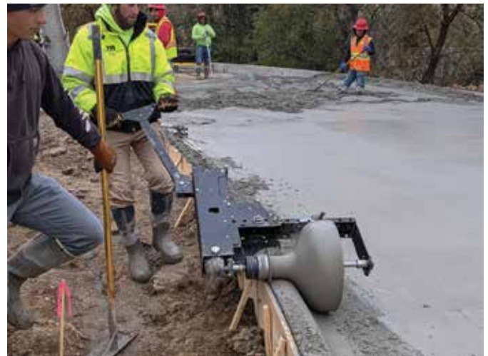
Walk-behind curbing machines with monolithic kits and battery-operated walk-behind curbing machines are two options that contractors may consider for a more streamlined process of hand-shaping curbs
