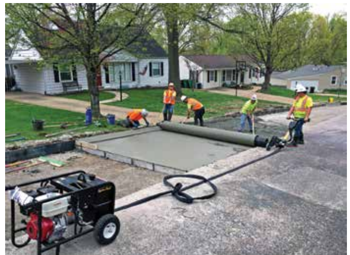
For some monolithic concrete placements, contractors may benefit from using one machine to simultaneously shape the curb and gutter and flatwork. This capability comes in the form of a custom drum with a hydraulic screed
