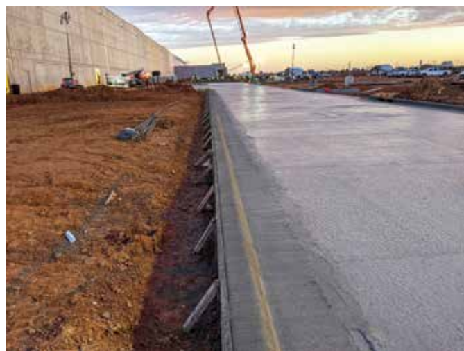
The monolithic placement process allows contractors to improve efficiency by completing flatwork and shaping the curb and gutter at the same time (all photos courtesy of Curb Roller Manufacturing)
