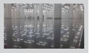
penetrating sealer that provides waterproofing and improves chemical resistance for the concrete. Its fast installation process can help contractors save weeks in construction schedules. In addition, this flooring solution enhances energy efficiency by maximizing light reflection, reducing the need for artificial lighting.
