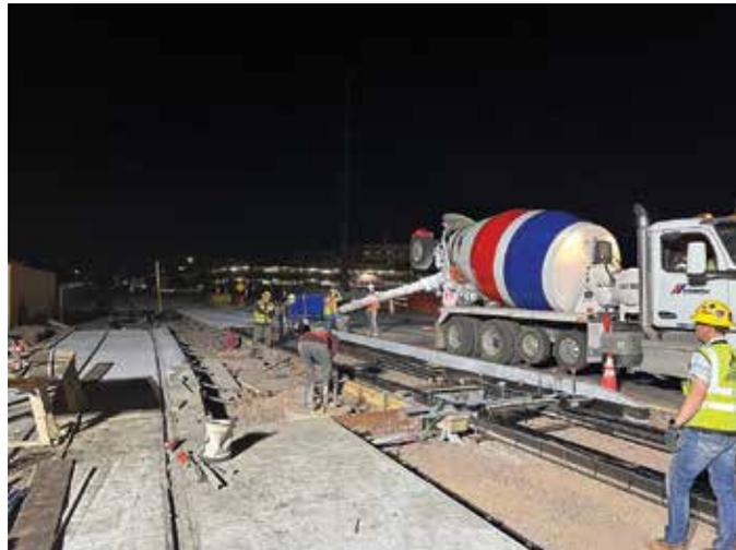
**Fiber-reinforced concrete placement of track slabs for Phoenix’s light rail extension**
