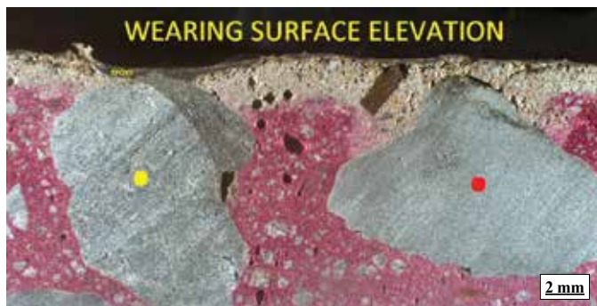
Fig. 3: A compromised wearing surface layer in a saw-cut surface of a scaled concrete core section following the application of the phenolphthalein. The cementitious constituents in the concrete are Type IL cement and fly ash, and coarse aggregate is a durable limestone rock
