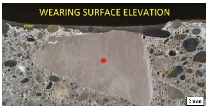
Fig. 4: A compromised wearing surface layer in a lapped surface of a scaled concrete core section. The cementitious constituents are Type IL cement and slag cement, and coarse aggregate is a limestone rock
