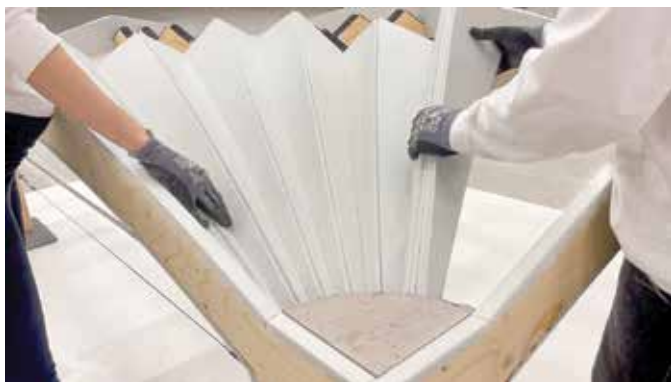
The plywood strips can be unfolded like a fan on site, causing them to bend into shape
