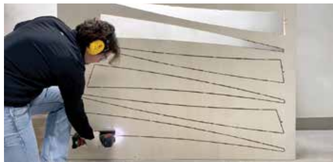
A plywood sheet is cut into individual curved strips
