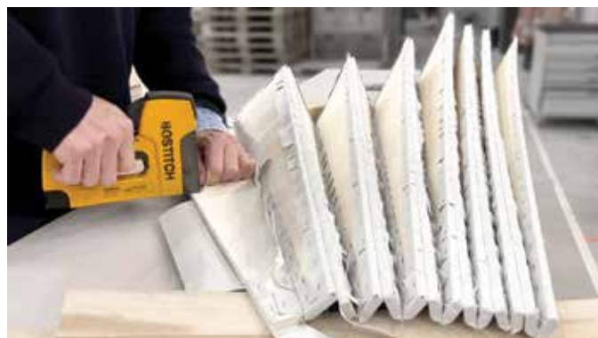
Textile layers are applied to one side of the strips to connect them
