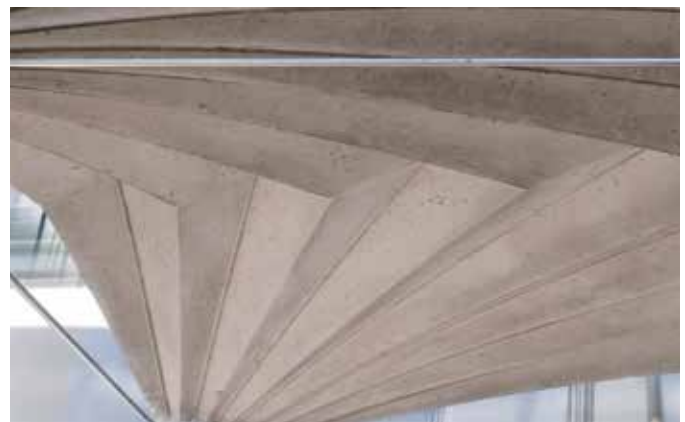
A structure after removal of the Unfold Form
