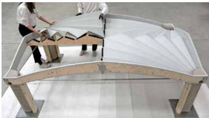
The four individual parts are joined to create the formwork, which has the capacity to hold up to a tonne (1.1 ton) of concrete
