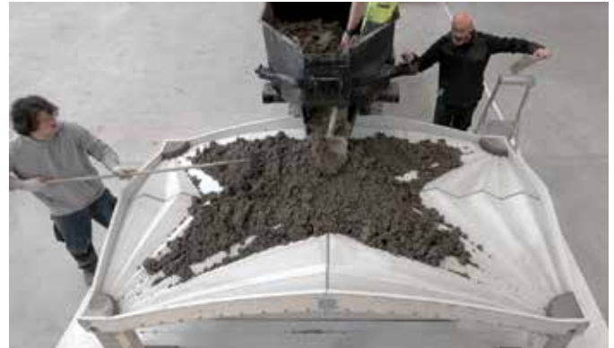
The concrete is placed directly onto the formwork. Once it has cured, the formwork can be removed from underneath
