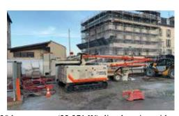
Power supply selections include a 50 horsepower (37,285 W) electric motor or a 30 horsepower (22,371 W) diesel engine with a soundproofing option. The arm folds up in a "z" formation to make the machine easier to haul on a trailer.
