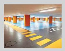
(41 and 50°F). The cured epoxy resin products are characterized by an aesthetic, glossy surface. Clouding, which is caused by haze formation, is avoided. This product creates color stability and is resistant to mechanical and chemical influences.
