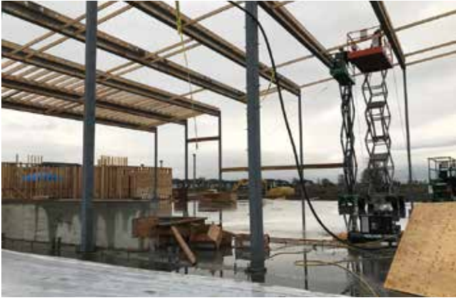
Fig. 1: SAY Health and Community Centre in Chilliwack, BC, Canada, during construction. The gymnasium's concrete floor included Hard-Cem for enhanced abrasion resistance
