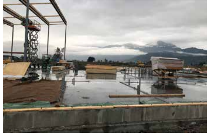
Fig. 1: SAY Health and Community Centre in Chilliwack, BC, Canada, during construction. The gymnasium's concrete floor included Hard-Cem for enhanced abrasion resistance
