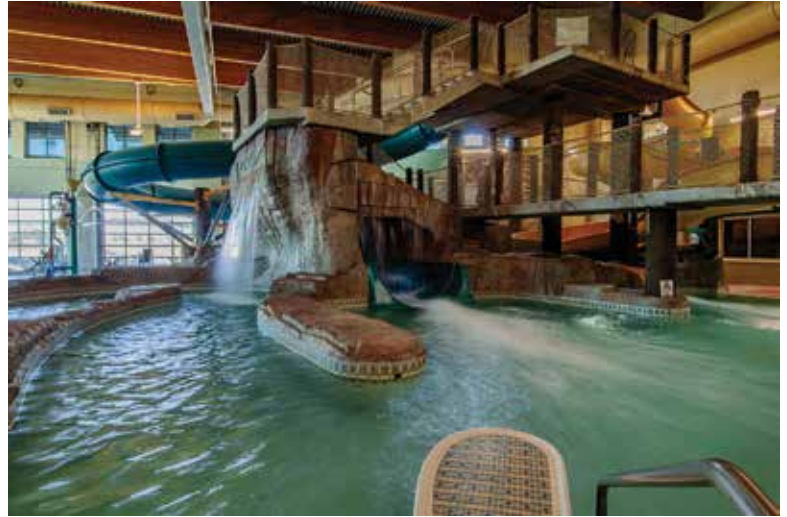
Paul Derda Recreation Center Revitalization
