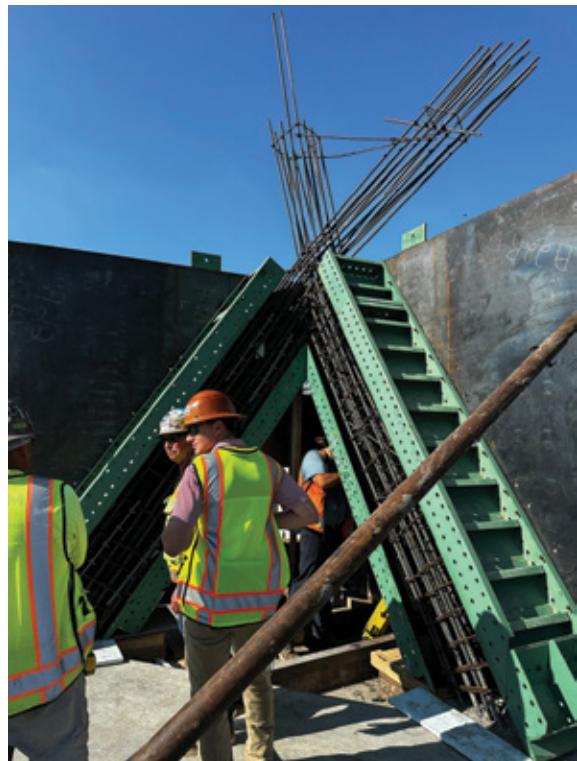
Fig. 5: Formwork for the corner columns being set in place
