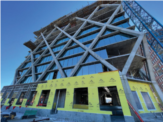
Fig. 1: Oblique view of the façade showing the façade slips behind the exterior diagrid column system
