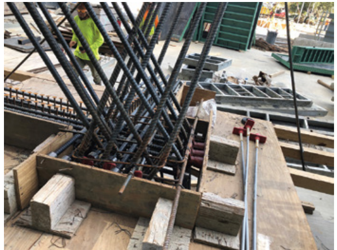
Fig. 4: Reinforcement mockup of the corner column/slab joint
