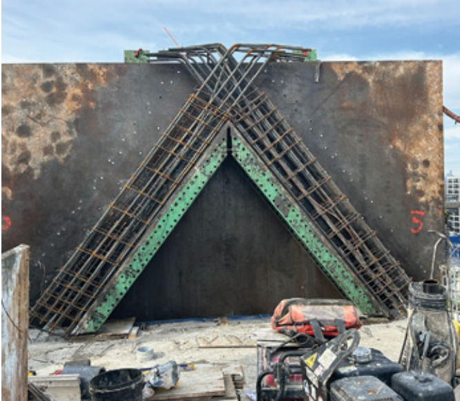
Fig. 6: Formwork for the edge columns at the rooftop
