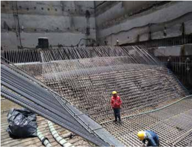
Fig. 5: Views of the mat foundation during construction (photos courtesy of Fernando Romo Consultores)
