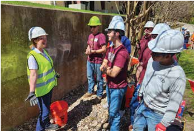
ACI Texas State University Student Chapter’s concrete repair project
