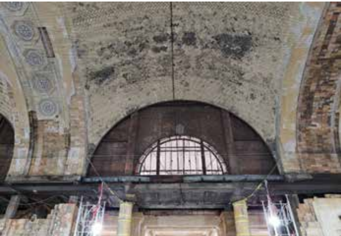
Before and after views of the Guastavino tile vaults at Michigan Central Station
