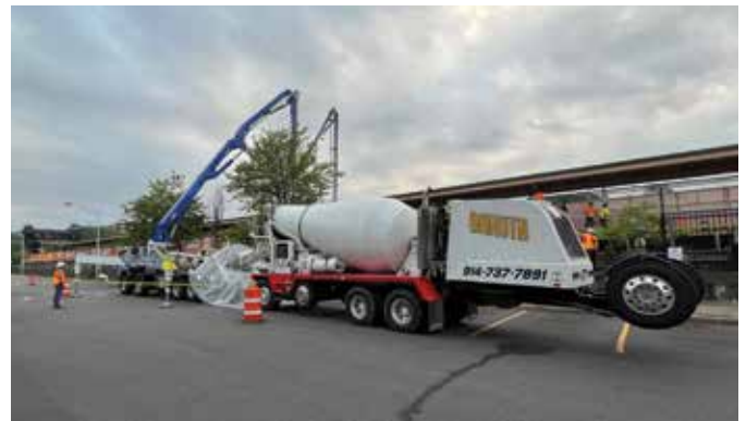
Thalle delivers concrete to Metro-North's Beacon Station
