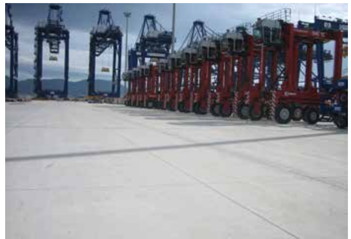
Fig. 1: Pavement with Type I steel fibers at the Maersk Container Terminal, Algeciras, Spain, constructed in late 1990s
