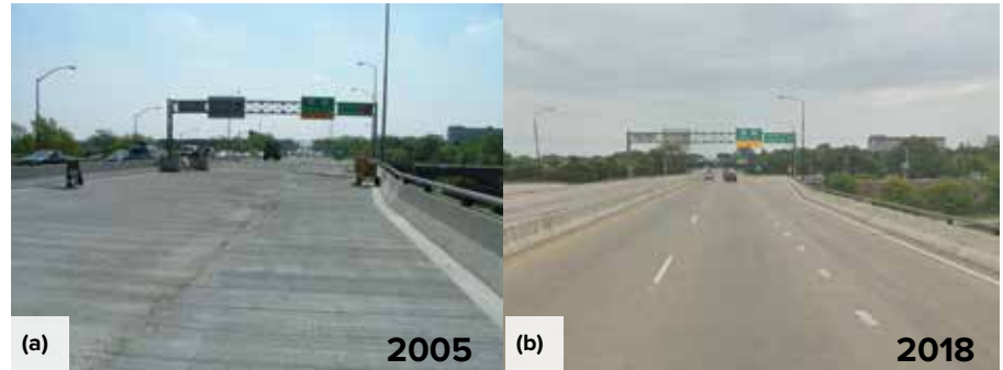
Fig. 3: Views of the deck of the Mason Street Bridge in Green Bay, WI, USA, which was constructed with synthetic macrofibers: (a) during construction in 2005; and (b) after more than 13 years of service
