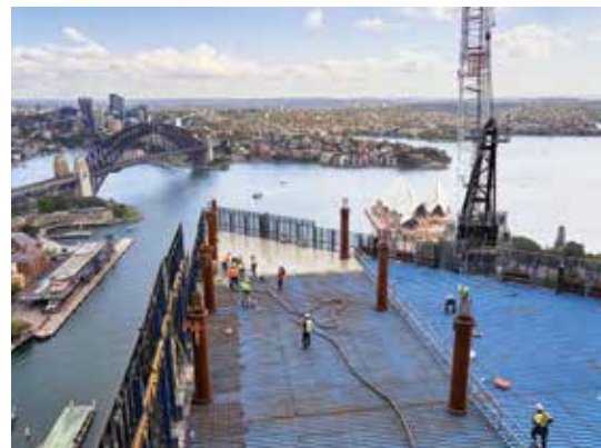
Quay Quarter Tower under construction
