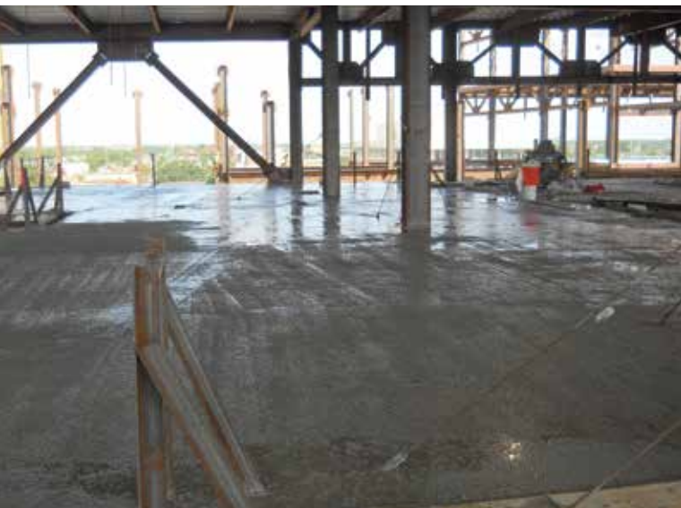
Bleed water coming to the surface prior to finishing (photo courtesy of Arcosa Lightweight)
