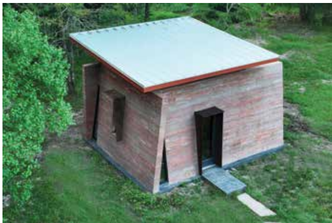
Fig. 4: Finished cabin with walls leaning at 8 degrees against each other on the corners like a house of cards
