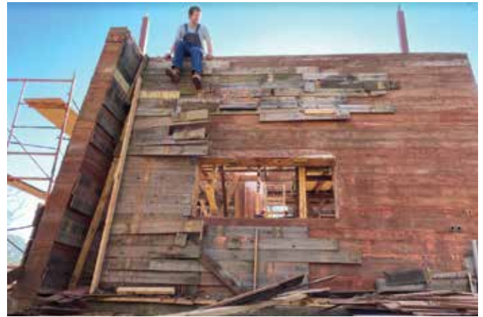
Fig. 3: Concrete walls were textured using boards salvaged from a barn
