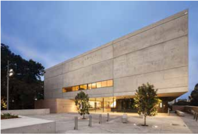
Chau Chak Wing Museum was designed as a cantilevered concrete box perched atop a glass and sandstone-colored precast podium
