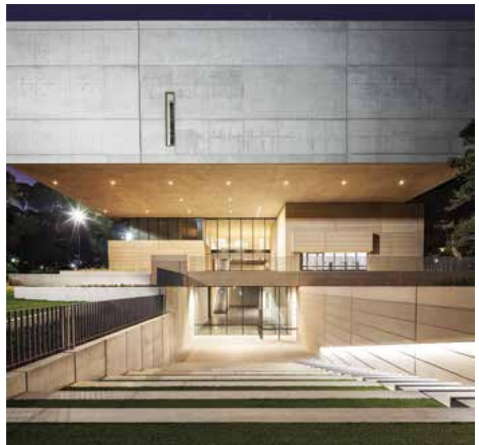
Project team architects Kiong Lee and Graeme Dix describe the museum as a direct expression of concrete as architecture, structure, and finish
