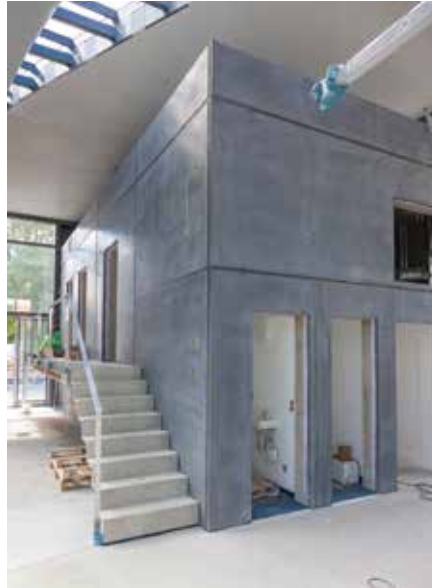
Fig. 2: The two-story box structure within The Cube is made of precast concrete insulated double walls; a section shown on the right by Manfred Curbach (photos courtesy of Stefan Groeschel, IMB, TU Dresden)
