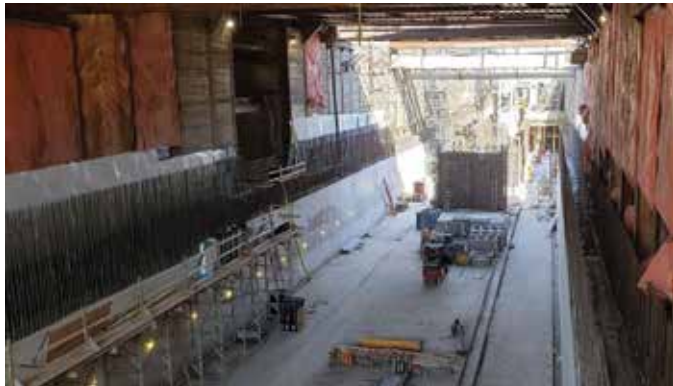
Fig. 2: Multiple mass concrete placements at Eglinton LRT Station
