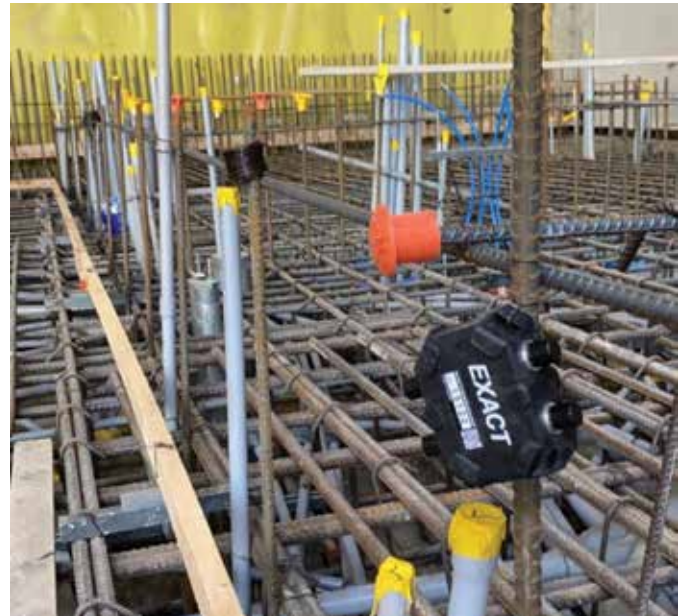
Fig. 3: Temperature monitoring equipment was installed shortly before concrete placement
