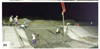
Fig. 8: Concrete placements at the JEC-FMC: (a) blinding layer in the sloped side; (b) a panel in the base slab; and (c) a panel at a sloped side
