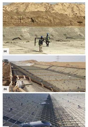
Fig. 7: The sloped sides of the JEC-FMC were tied to the base slab using bespoke splice bars: (a) a worker carries a bundle of splice bars; (b) prior to concrete placement, an overview of an upstream section of the JEC-FMC, showing grids, weep holes, and channel edge formwork; and (c) detail of lap splice at base-slope intersection
