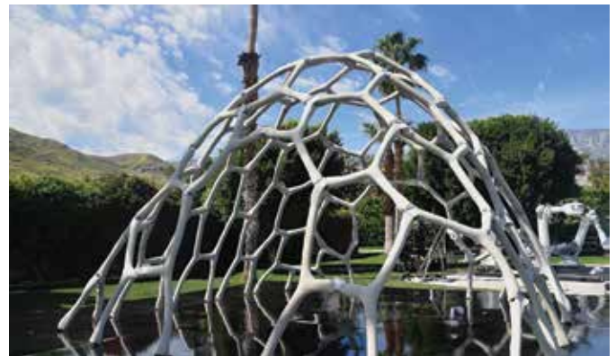
Fig. 8: The Mars Canopy was constructed without reinforcing bars 20
