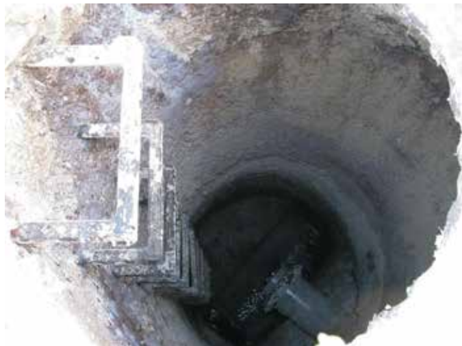
Fig. 2: Calcium sulfate (gypsum) forms a whitish foamy mass on concrete
