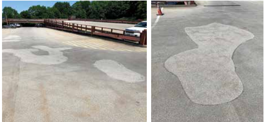
Fig. 7: A parking garage deck in Utica, NY, USA, repaired with the rubber-modified repair material, after 4 years in service
