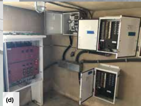
Fig. 6: ICCP system features: (a) anode and isolation from low-cover reinforcing bar; (b) grouted anode slots; (c) balcony deck as finished with vertical conduit (photo taken 2010); and (d) control and power system components (May 20, 2019)
