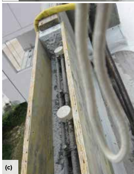
Fig. 5: In-progress repairs: (a) exposed reinforcement in corridor; (b) exposed reinforcement in parapet; and (c) GCP and formwork installed at parapet repair
