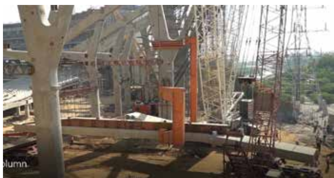
Fig. 9: An HY column is lifted by two cranes
