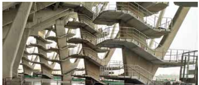
Fig. 15: Vomitory staircases at HY columns
