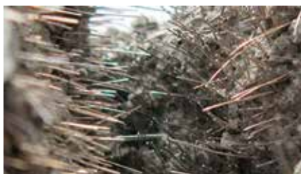
Fig. 3: Fractured surface of a UHPC structural member with visible fiber pullout
