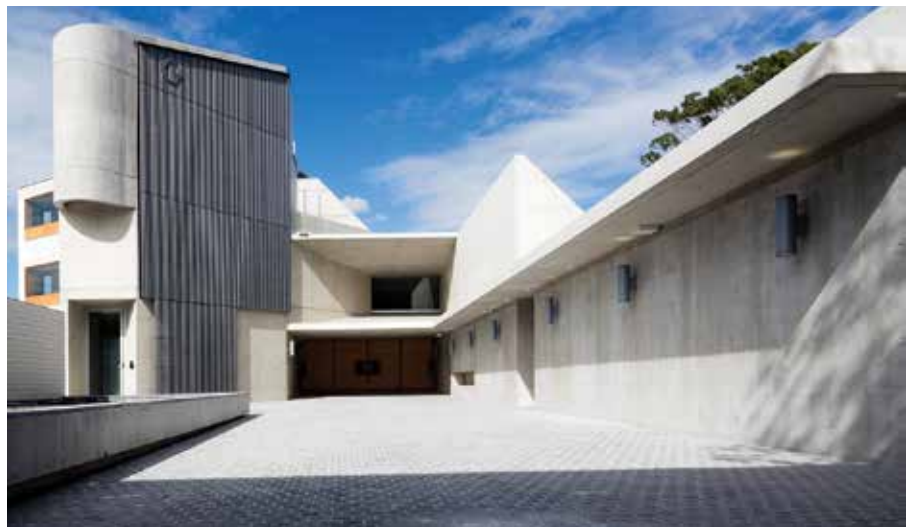
Fig. 1: Punchbowl Mosque, Sydney, Australia, with main entry doors facing the street and a single minaret adjacent to the entry (left) (photo by Brett Boardman, courtesy of Candalepas Associates)
