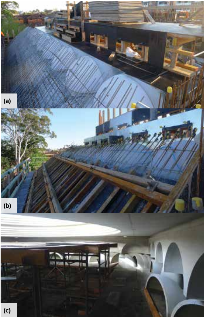
Fig. 4: Muqarnas were formed using molded fiberglass minidomes spaced 120 mm (5 in.) apart, and the flat surfaces between minidomes were formed using galvanized steel on plywood panels: (a) view of minidome forms installed on scaffolding; (b) view of exterior formwork for the sloping roof; and (c) view of minidomes during stripping operations (photos by Adrian Curtin, courtesy of Boral Australia)
