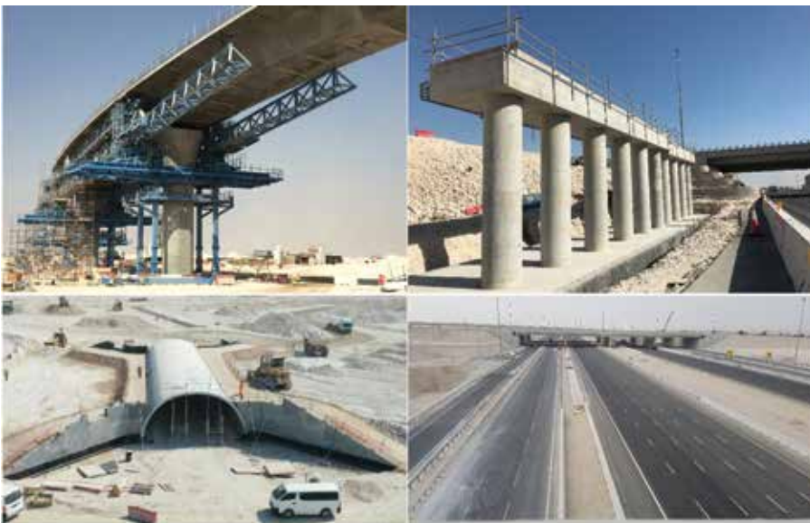
Fig. 2: Typical structures of the New Orbital Highway Contract 3 project
