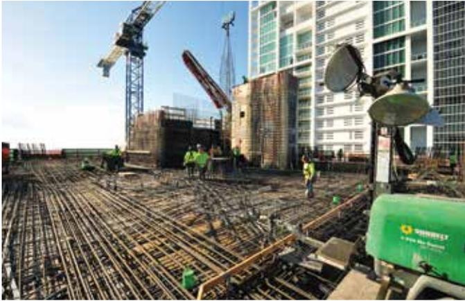
**Fig. 4:** Column-free floor plates were created using post-tensioned, 11 in. (280 mm) thick slabs (photo courtesy of Plaza Construction)
